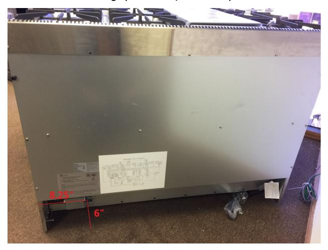
Distance from inlet gas pipe to right side of the range is 8.25".
